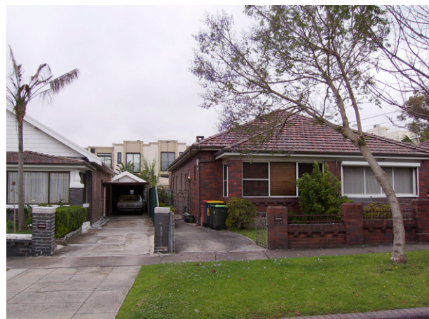
Figure 34.12. Although most of these houses were built originally with an open front porch these have been enclosed to provide additional living space over the years. The houses on this side of the street are set well back, providing space for a generous front garden. Access is still on the side elevation but a more formal porch has been provided in most cases. Windows are sash-framed which is typical of the style.
