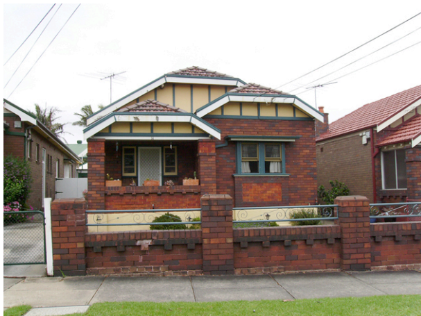
Figure 34.5. to 34.9 Although the half gabled roofs create an unusually distinctive streetscape the houses themselves modest in scale and form, with their front door located on the side elevation and the small porch accessed from the interior only. This has facilitated their enclosure to provide additional living space. The decorative brickwork inlaid to decorate the facades can also be seen in this photograph.
